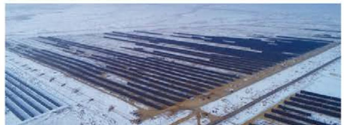
Vertex modules in extreme cold weather (Image: Trina Solar)
